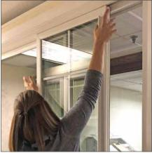
STEP 5: Remove the left sash by pulling down on both tilt latches and pulling the top of the sash inward.
