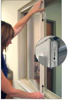
STEP 3: Release the left sash by pulling both tilt latches (top and bottom) toward the center of the window and swinging the sash in.
