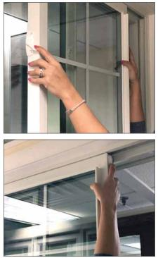
STEP 3: Simultaneously rotate the cam lock to the wash position (left) while depressing the tilt latch on the right.
