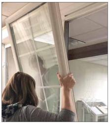
STEP 4: While holding the cam lock in the wash position and depressing the tilt latch, pull the top inward.
