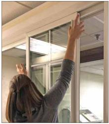
STEP 5: Remove the left sash by pulling down on both tilt latches and pulling the top of the sash inward.
