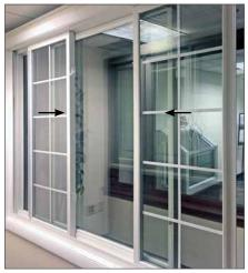
STEP 2: Unlock and open both sashes so there are equal openings at either end.
